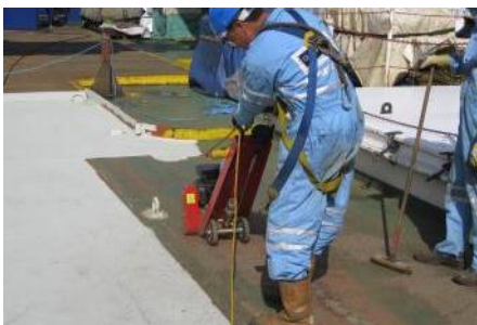
Coating & corrosion removal
